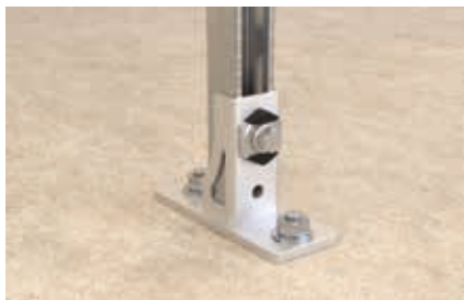
Channel installation at the wall
