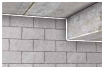
Joint de construction
